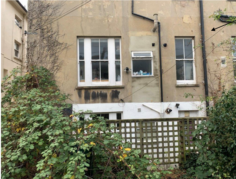
Rear of No. 45 Clarendon Villas
