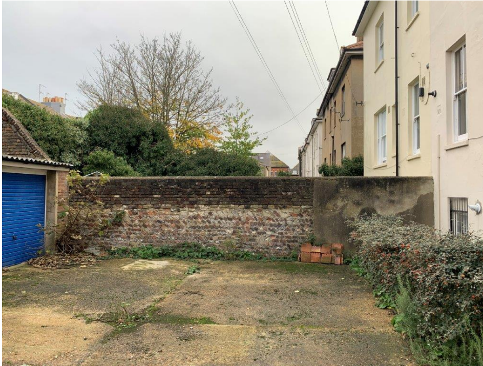
← Rear of No. 43 Clarendon Villas
